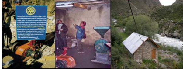
Jang MHP power house
