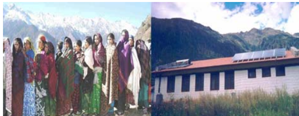
Solar system Simikot hospital
